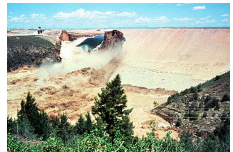
Failure of Teton Dam, USA (5 th June 1976)
